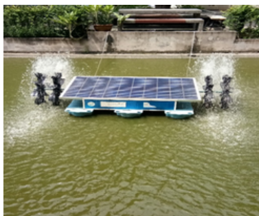
Main combine sewerage pond at KMUTNB Bangkok Campus with the solar power turbine
