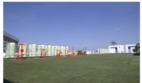
Rainfall water storage tanks on the upper deck level
